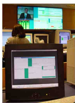
CommandaNT window manager using touch screen solution.
